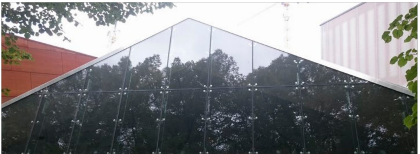
Otaniemi subway station, Helsinki – strength analysis of the façade with glass fins, and fixing accessories
