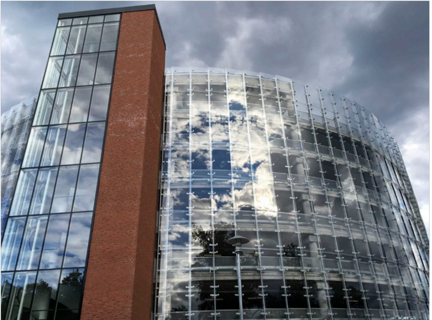
Solna parking house, Stockholm – facade point fixings
