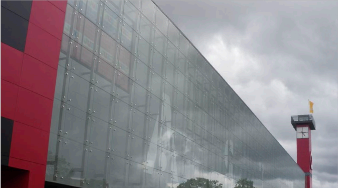
Astri Shopping Centre, Narva – facade point fixings and spider-fittings
