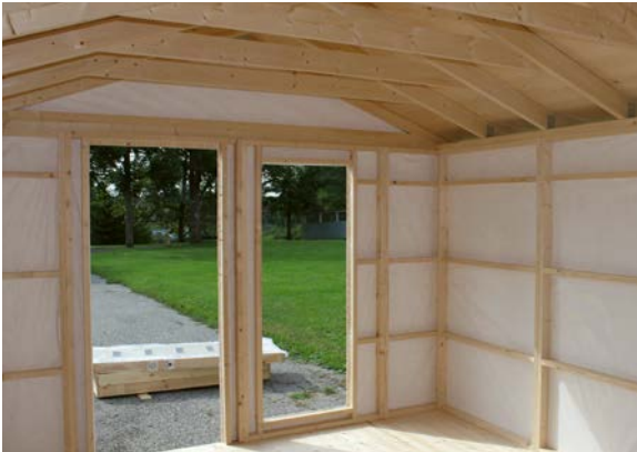
Internal view, walls covered with wind-protection plastic
